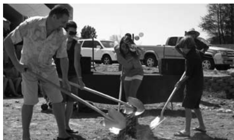
With help from UP, the Cader Family broke ground to rebuild after a 2007 wildfire.
